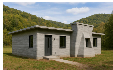
3D concrete-printed floodbuster home
